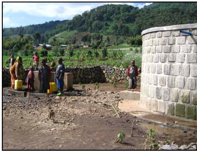
Figure A-8: New community water tank from Bunyenyeri source
