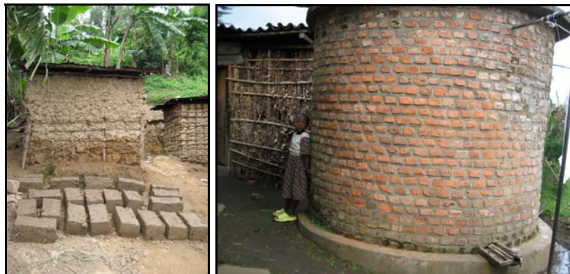
Figure A-11a & b: Recently made compacted bricks and baked-brick water tank (photographs by D. Cresti and author)
