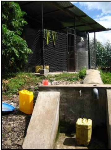
Figure A-6: New trackers' house tanks
