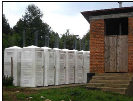
Figure A-10: New toilets at primary school
