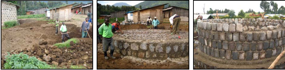
Figure A-9: Progress of Bushokoro community water tank
