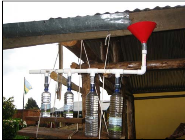
Figure 3-10: CL array on new iron roof
